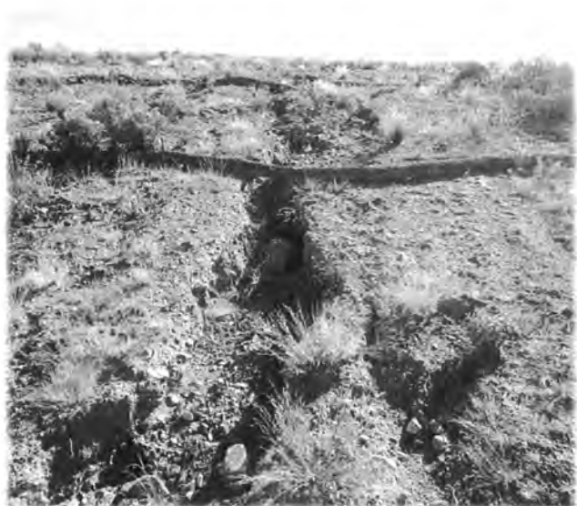
PHOTOGRAPH NO. 12 Erosion rills parallel to the west spillway. Viewed from the North.
