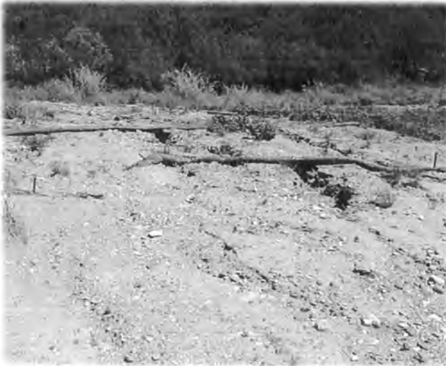
PHOTOGRAPH NO. 5 Erosion rills located on north end of west slope. Viewed from the east.
