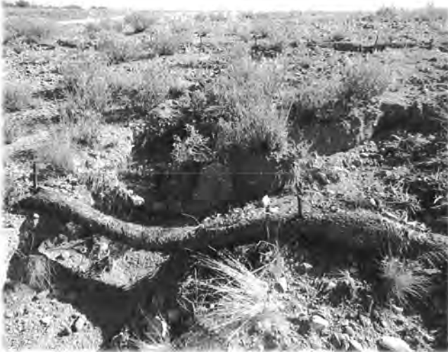
PHOTOGRAPH NO. 9 Erosion rills located on north slope. Viewed from the west.
