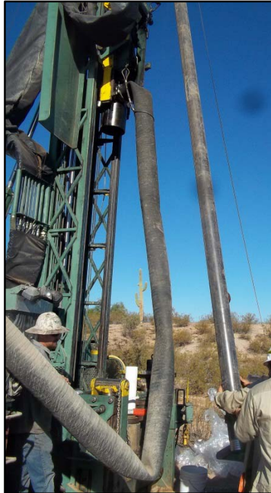
Factory sealed, 5-inch, Schedule 80 PVC well casing and well screen with 0.040-inch horizontal slots.
