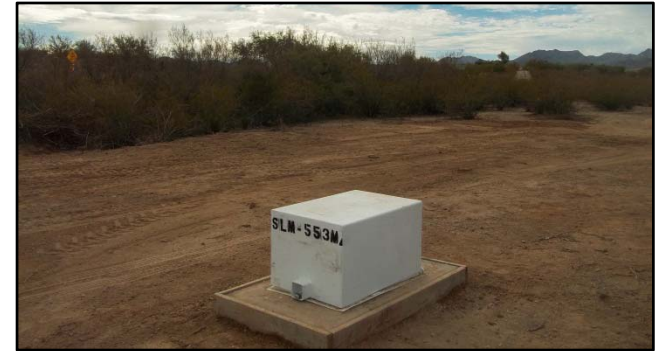
Above ground, Tucson Vault Surface Completion
