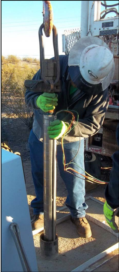
Grundfos 10Hp Test Pump, lowered with 2-inch steel drop pipe.
