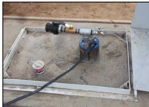
1-inch galvanized steel drop pipe; Sounding tube is 2-inch Schedule 40 PVC with 0.010-inch horizontal slots from 310-320 feet bls with a PVC end cap.
