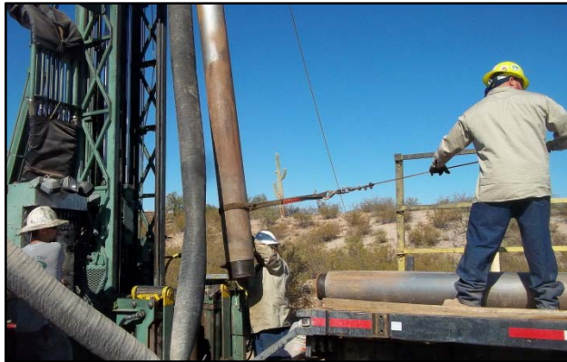
Dual Wall 10 3/4-inch outer diameter drill pipe.
