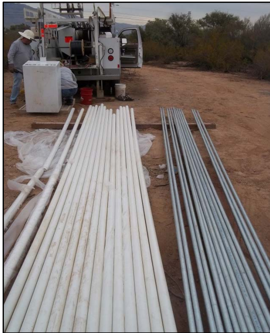
1-inch galvanized steel drop pipe; Sounding tube is 2-inch Schedule 40 PVC with 0.010-inch horizontal slots from 310-320 feet bls with a PVC end cap.
