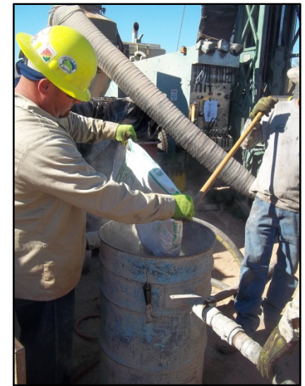
Annular materials included hydrated bentonite pellets, 8-12 mesh sand, #60 (fine) sand, bentonite grout and cement grout, which were gravity fed between the drill pipe and the well casing.
