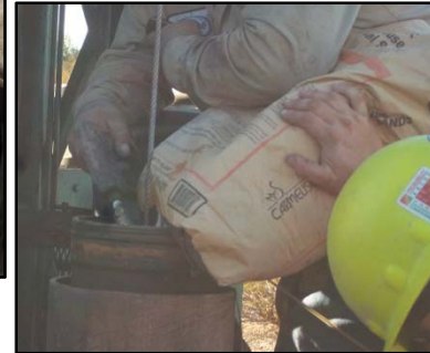
Annular materials included hydrated bentonite pellets, 8-12 mesh sand, #60 (fine) sand, bentonite grout and cement grout, which were gravity fed between the drill pipe and the well casing.
