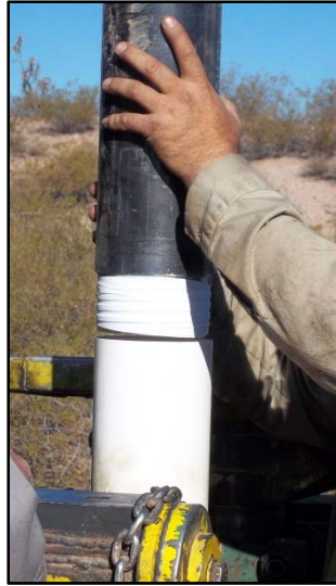
Factory sealed, 5-inch, Schedule 80 PVC well casing and well screen with 0.040-inch horizontal slots.
