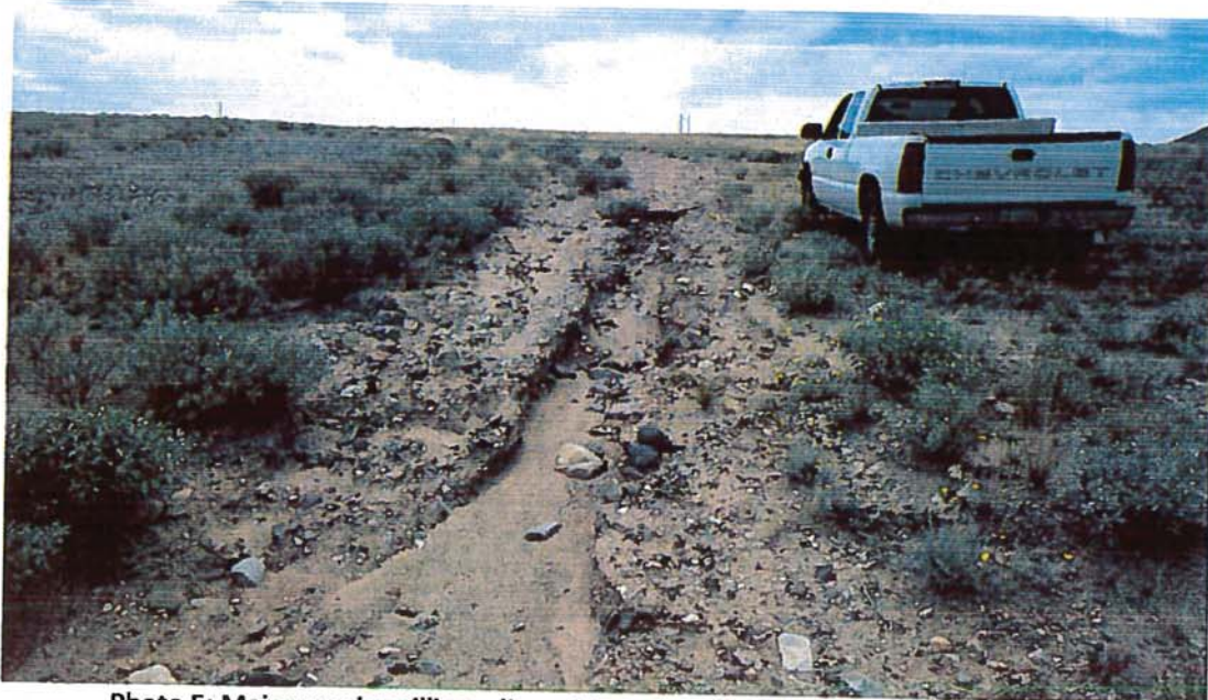
Photo 5: Major erosion rilling adjacent to rock spillway, north central landfill cap
