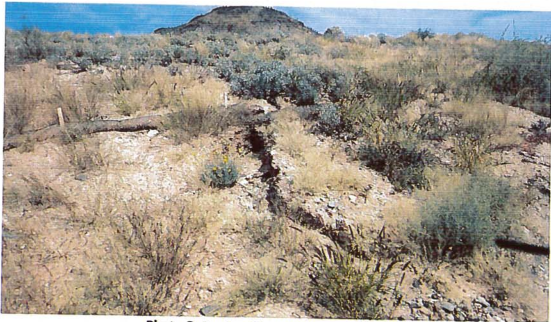
Photo 8: Erosion rill on south slope of landfill
