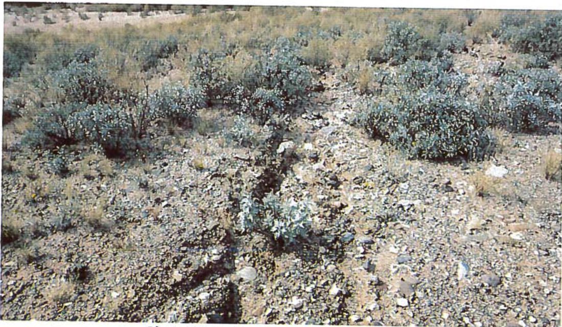
Photo 10: Erosion rill on west slope of landfill
