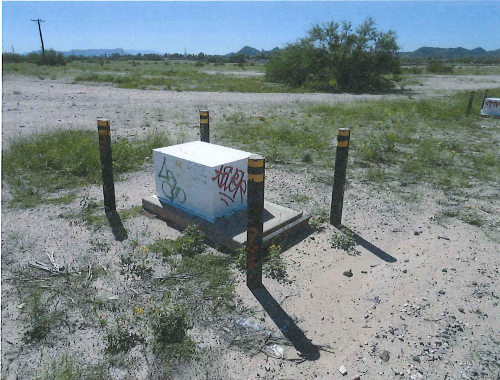
Photo 5: Graffiti on groundwater monitoring well
