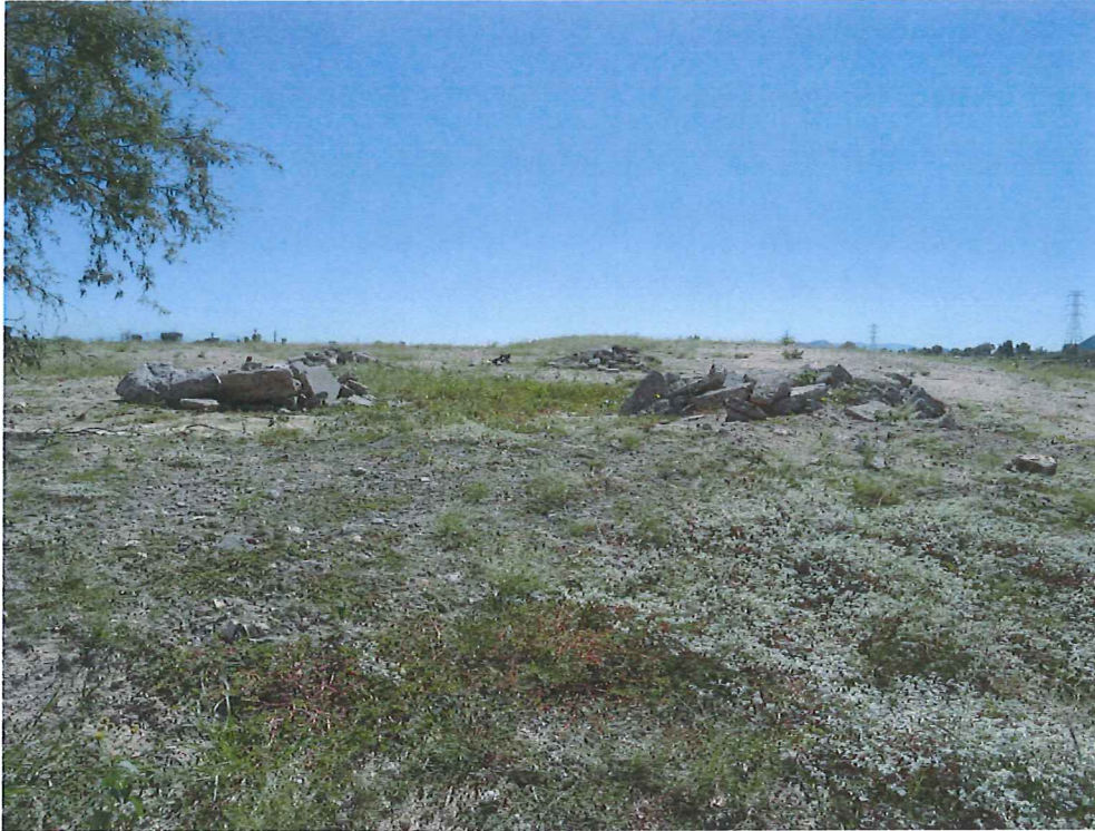
Photo 7: Concrete debris on landfill cap
