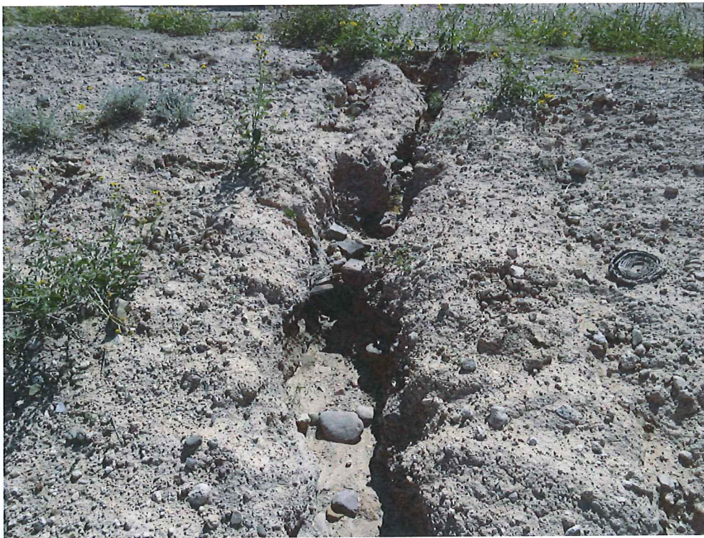
Photo 2: Exposed trash in rill on north landfill slope
