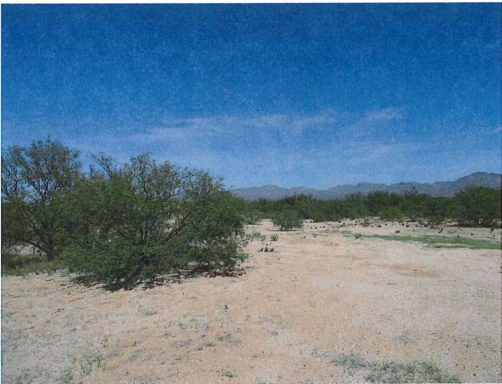
Photo 2: Ryan Airfield Landfill earthen cap, view to the NE
