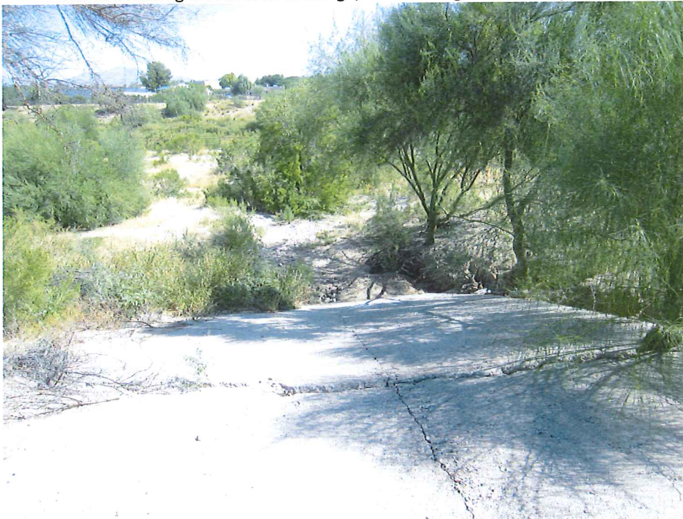
Photo 4: Lower portion of main drainage
