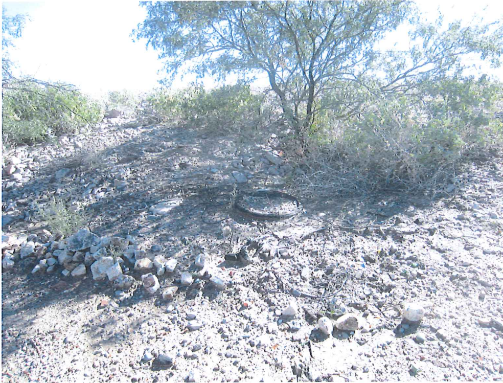
Photo 5: Exposed trash on slope adjacent to Mission Gardens
