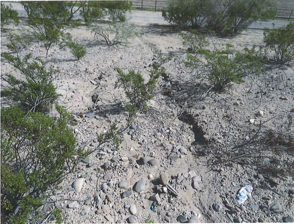
Photo 3: Rill erosion on east slope of landfill above County multi-use path
