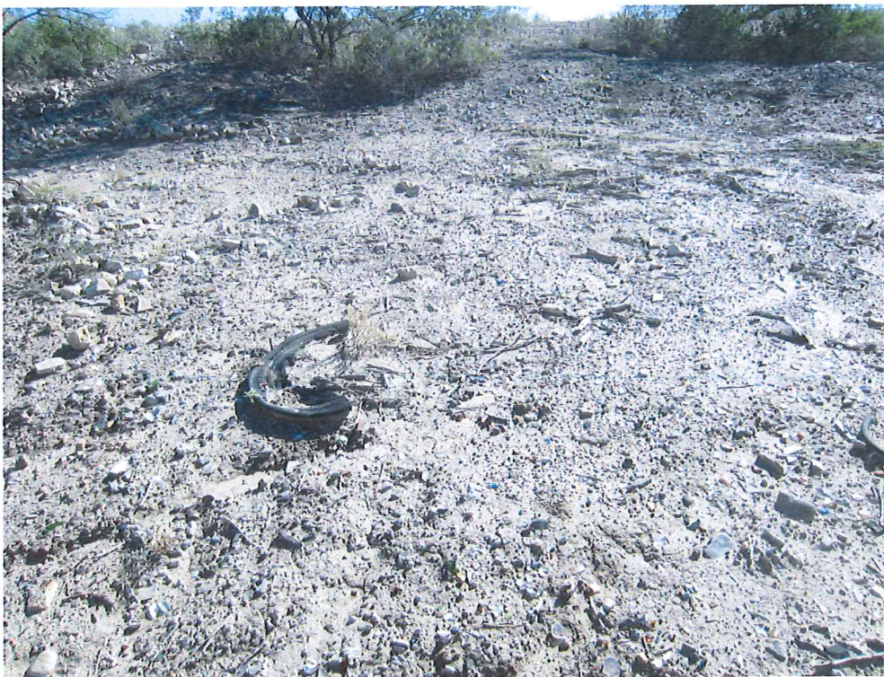
Photo 6: Exposed trash on slope adjacent to Mission Gardens
