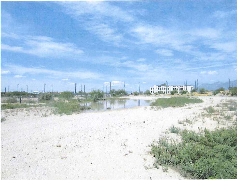
Photo 3: Ponding water on Congress Landfill
