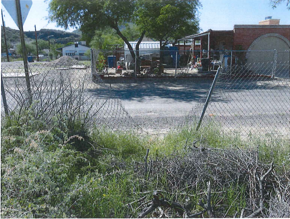
Photo 1: Fencing on northwest boundary of Nearthmont LF
